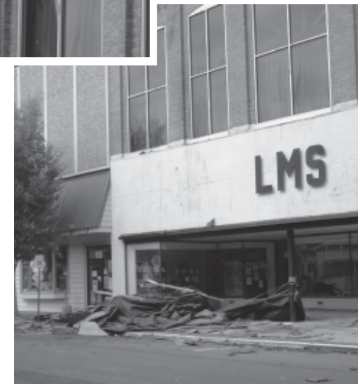
The center also experienced water damage.
