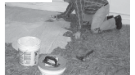
Bob Schwarz spreads tile adhesive in preparation for final step.
