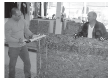
Jaime Jaseph (l) and Bob Kraft prepare flooring panel.
