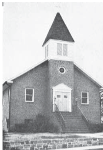
Holy Nativity Church Linden Avenue, Arbutus Supplied LMS with a Vicar while LMS assumed direction of church during 1941-43
